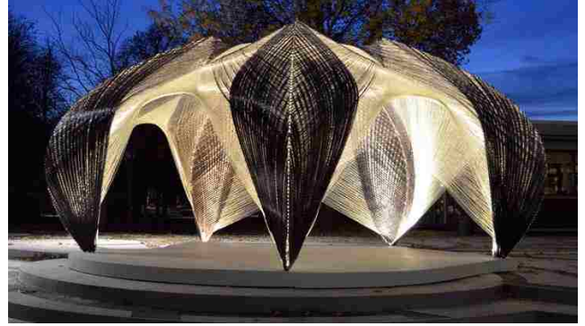
fig. 23 Monocoque carbon and glass fiber shell
